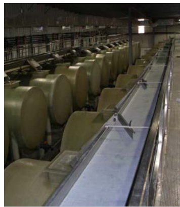
OLIVES OXIDATION SYSTEM FOOD TRANSFER PUMP
